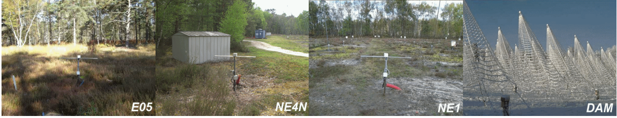
Figure 2: Some currently used active dipole antennas of the CODALEMA setup. From left to right : in a clear environment, close to a metallic shelter, in the center of the DAM, and a picture of the DAM itself.
